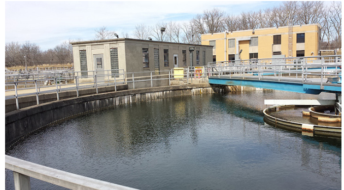
The City of Muncie Wastewater Treatment Plant
