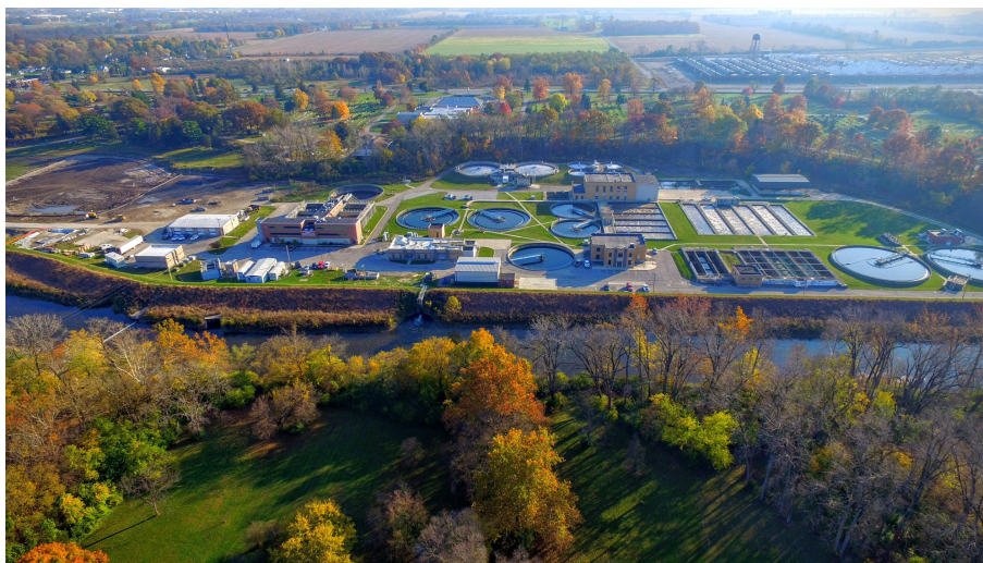
The 24 MGD Muncie activated sludge wastewater treatment plant serves a population of approximately 31,000.
